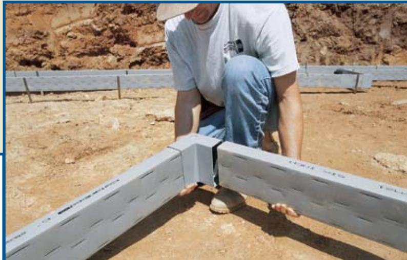
**Lineal sections, couplings, and corners ensure precise form set-up.**
